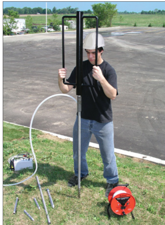
Installing Piezometers with a Manual Slide Hammer
